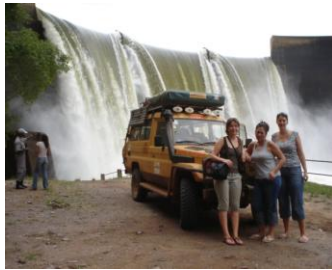
Cambambe Dam Wall
